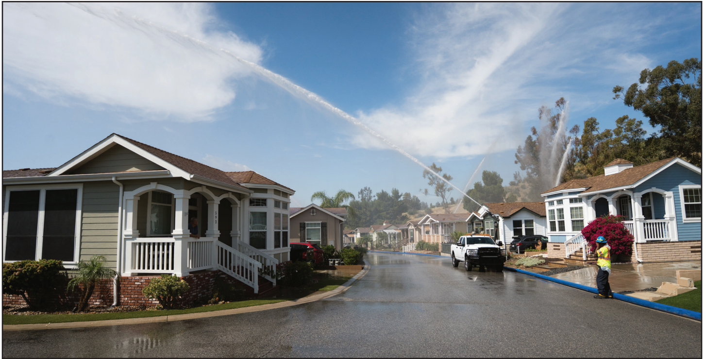
Inside Oakridge Mobile Home Park during the demonstration on March 24. A total of 63 pre-positioned high-capacity monitors with a 450-foot reach provided water coverage across all 600 homes in the park.
