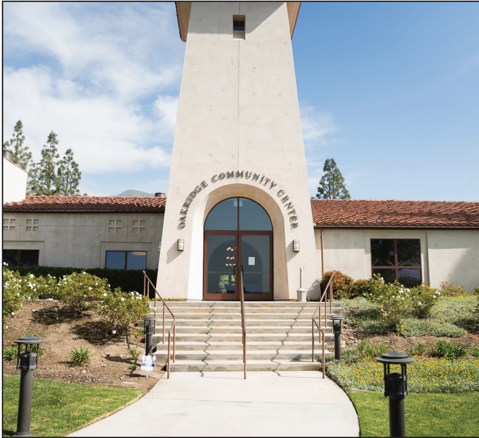
View of the front of Oakridge Mobile Home Park's Community Center.
